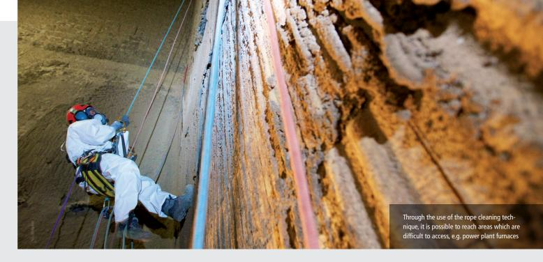
The cleaning specialists use the so-called rope-aided cleaning technology. This term is used for all rope-aided work carried which is out on structures or buildings that are difficult to access, e.g. radio towers, silos or industrial plants. Each climber is protected by two separately secured
