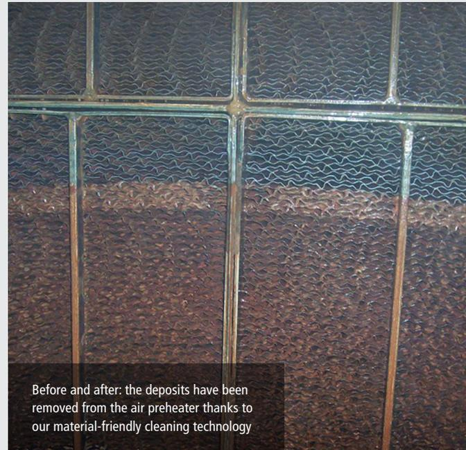
Before and after: the deposits have been removed from the air preheater thanks to our material-friendly cleaning technology
